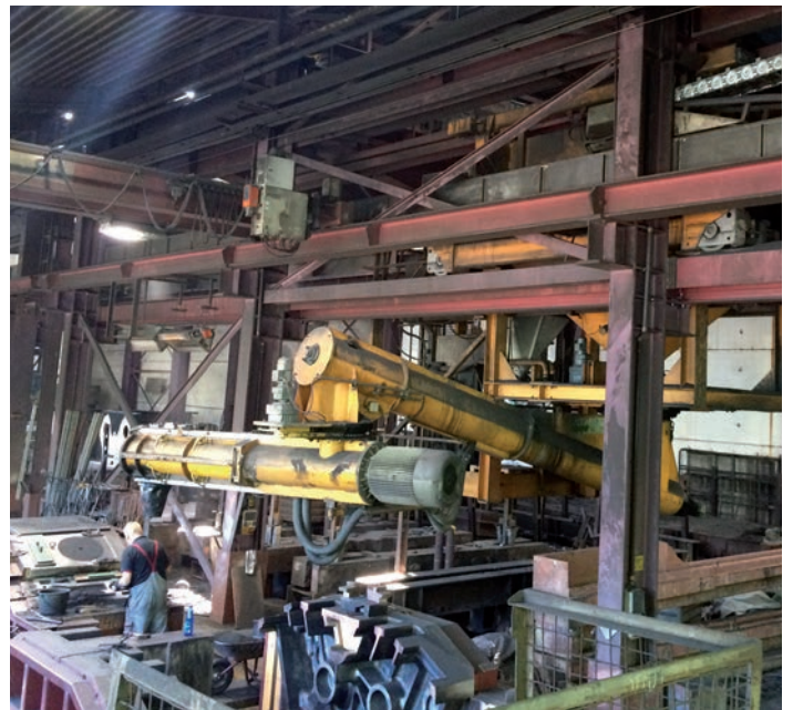
Insight into the casting house
